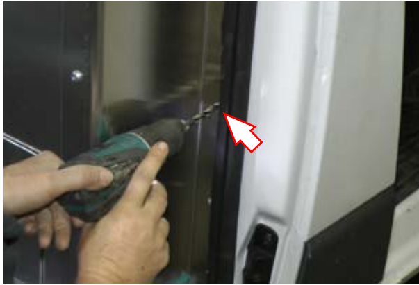
3/8" hole drilled in B-pillar
